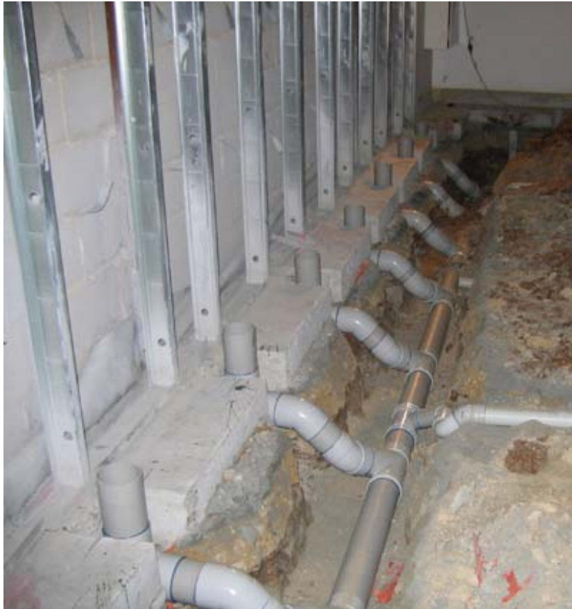
Rectification with 45° junctions
